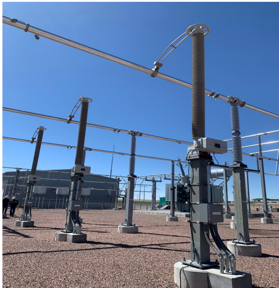
RCVT with High Accuracy Harmonic Measuring Capacity - ARM Reactor in Background
