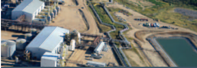
MEG Energy Christina Lake SAGD Post-Combustion CO 2 Capture Alberta, Canada
